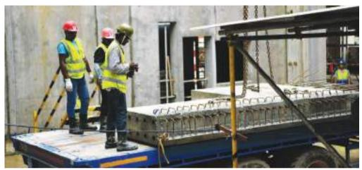
Precast components are RFID-tagged for individual tracking
