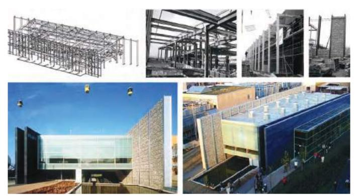
The Irish Pavilion: A steel structural frame with modular cladding that can be bolted together and taken apart
